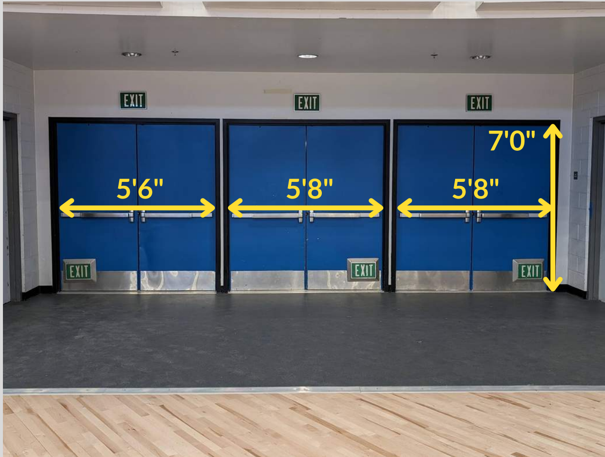
Exit Doors (3 double doors)
