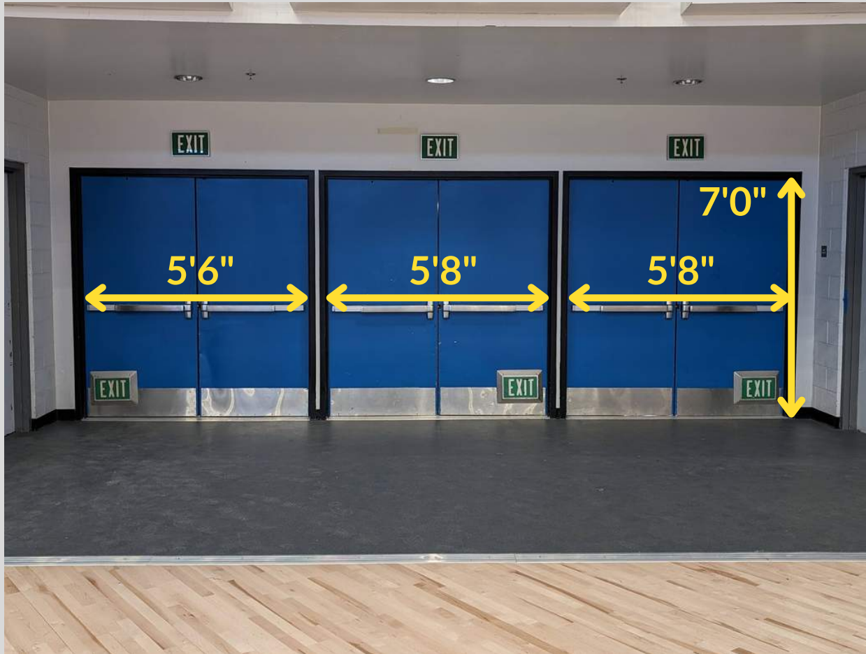
Exit Doors (3 double doors)
