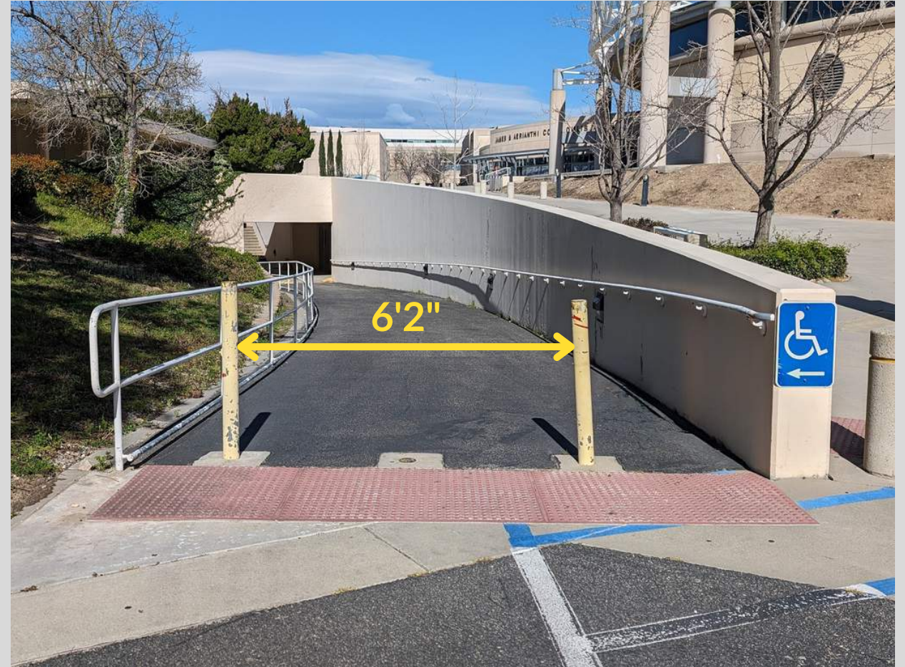
Ramp to Performance Entry
