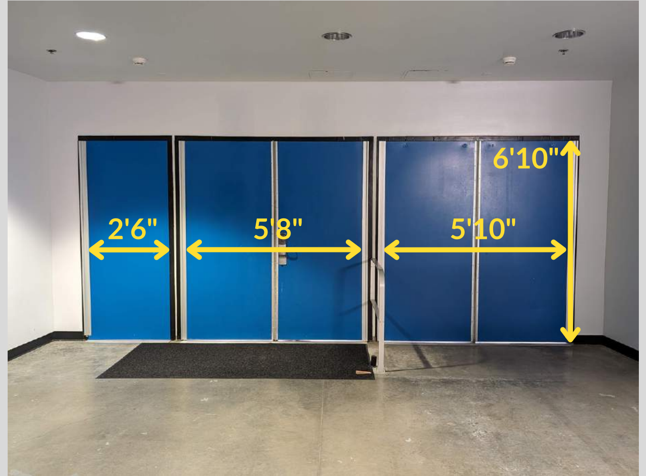
Entry Doors (1 single door; 2 double doors)
