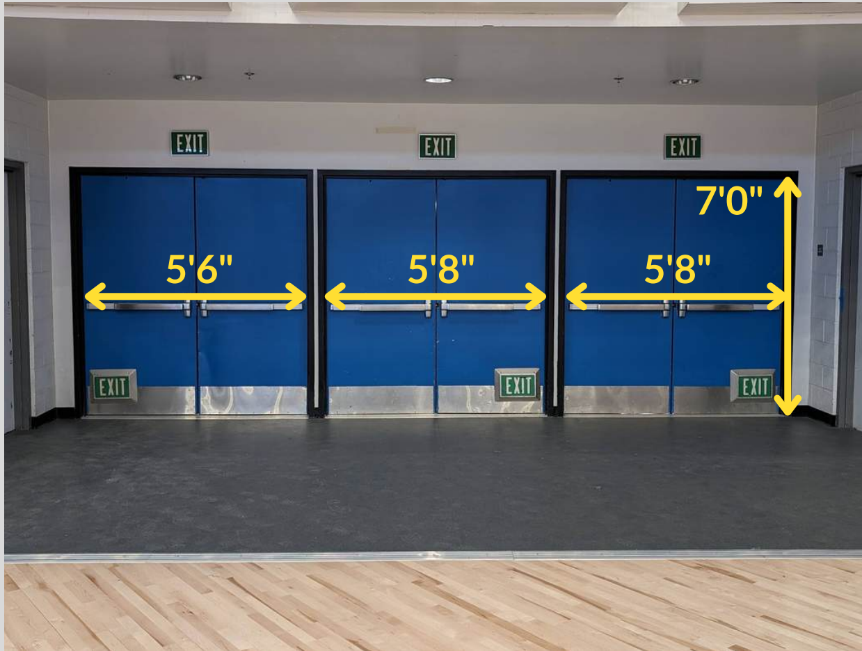
Exit Doors (3 double doors)
