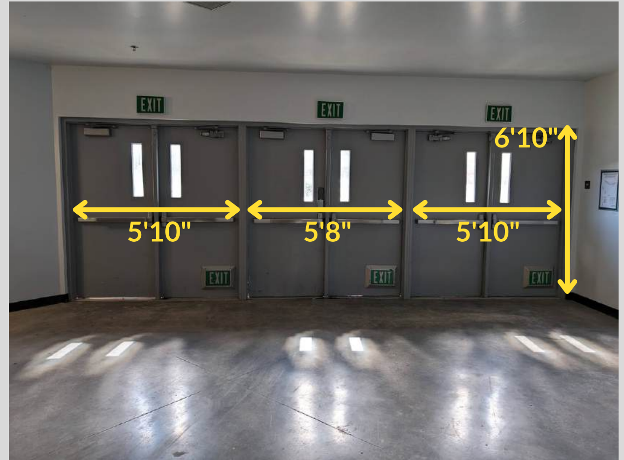
Exit Doors to Floor Folding (3 double doors)
