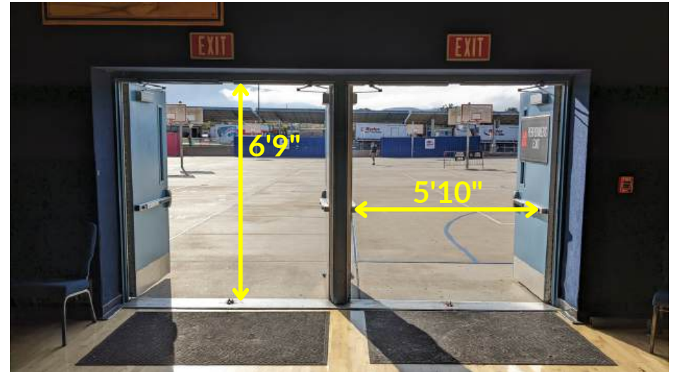
Exit Doors (2 double doors)
