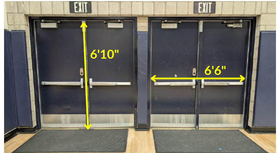
Exit Doors (2 double doors)
