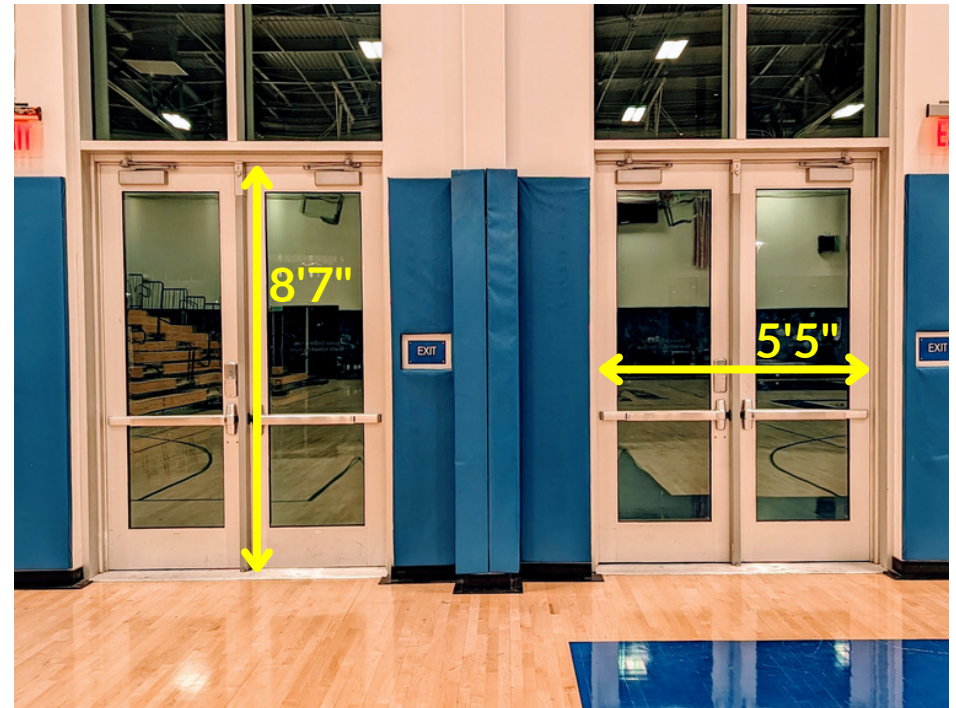
Exit Doors (2 double doors)
