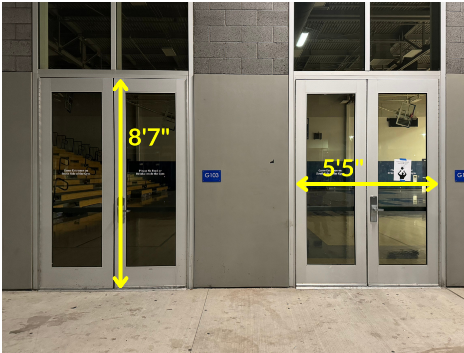
Entry Doors (2 double doors)
